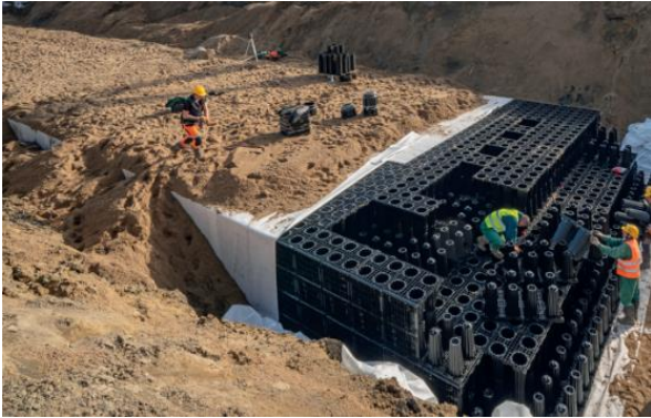
Figure 6 Honeycomb infiltration blocks installation (ACO Stormbrixx)
