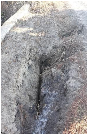
Figure 11. Concrete tympanum detached from the bridge superstructure - Photo by Marin Ilca
