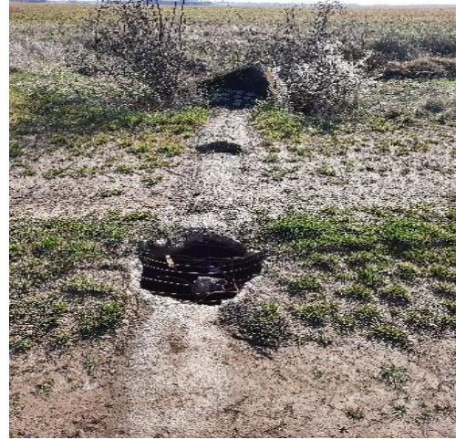
Figure 13. Corroborative factors that led to the destruction of the intubated passage (incorrect assembly and material wear) - Photo by Marin
