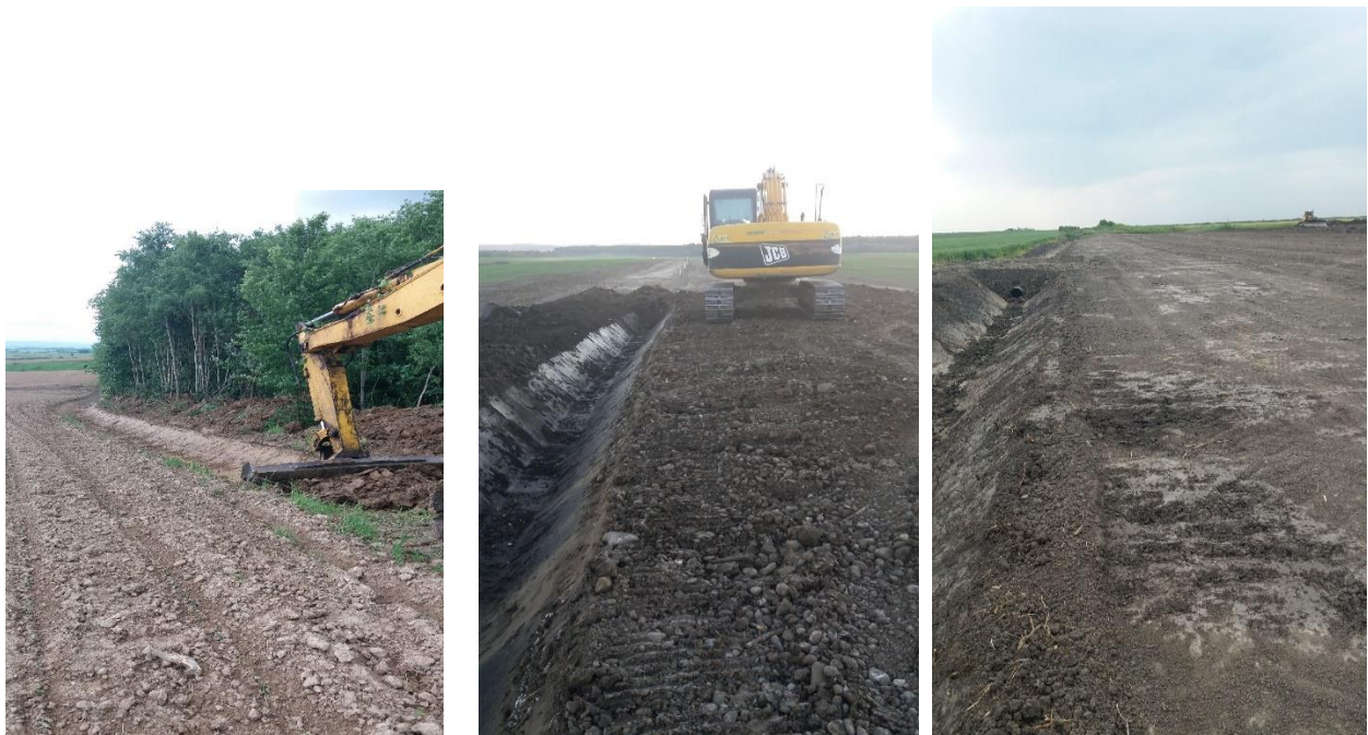
Figure 6. Digging ditches using the profiled bucket - Photo Marin Ilca
