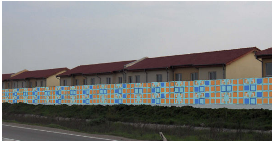
Fig. 6. Sound absorbing panels used in outdoor environment to protect residential areas.
