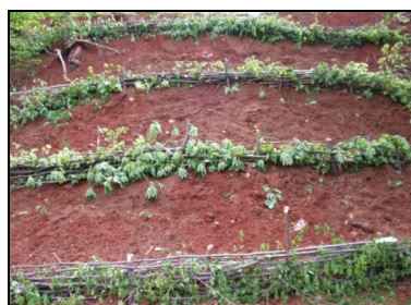
Fig. 2. Mattresses after the final step 2004) from the former bauxite quarry from Zece Hotare, Bihor
