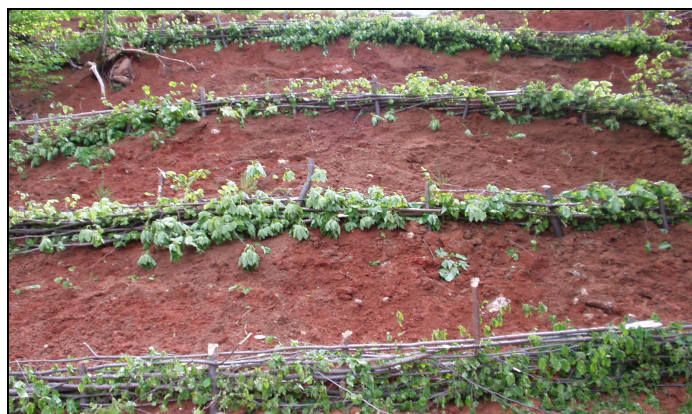
Fig. 3 Mattresse made of beech, after execution (2004), at the former bauxite quarry at Zece Hotare, Bihor
