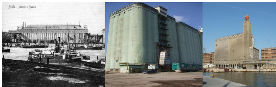
Figure 5. Reinforced concrete silos in Braila, Codlea and Pireus ports
