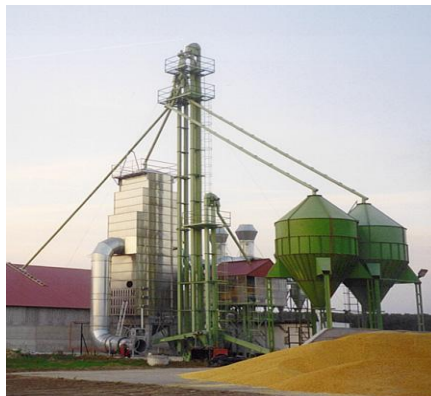
Figure 4. Reinforced concrete platform for grain storage in Biharkeresztes
