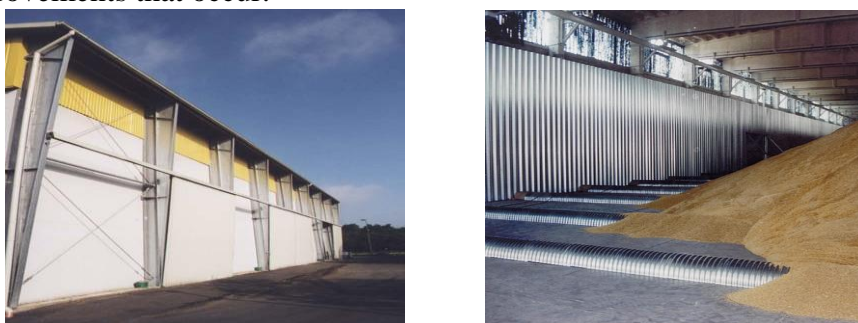
Figure 5. Warehouse made from panels and equipped with air circulation channels
